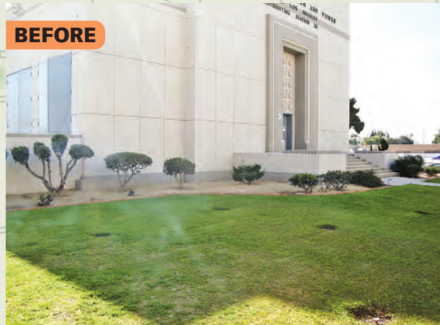
Distribution Station 28 West Los Angeles
