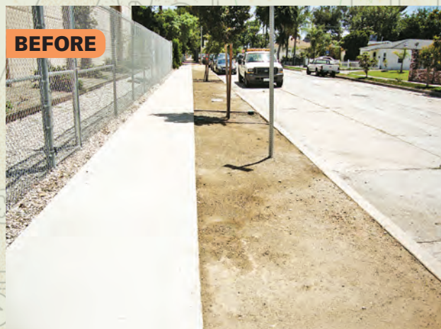
Distribution Station 85 Tujunga
