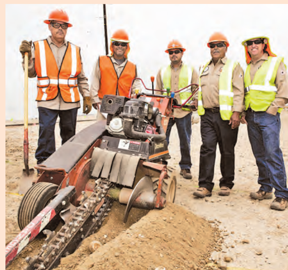
Digging an irrigation trench at the Sylmar Reservoir facility are (from left) Juan Raygoza, Gardener/Caretaker, 10 years of City service; Reyes Nuñez, Gardener/Caretaker, 6 years; Rodrigo Mendez, Capital Projects, 8 years; David Garibay, Gardener/Caretaker, 29 years; and Joseph Sanchez, Sr. Gardener, 7 years.
