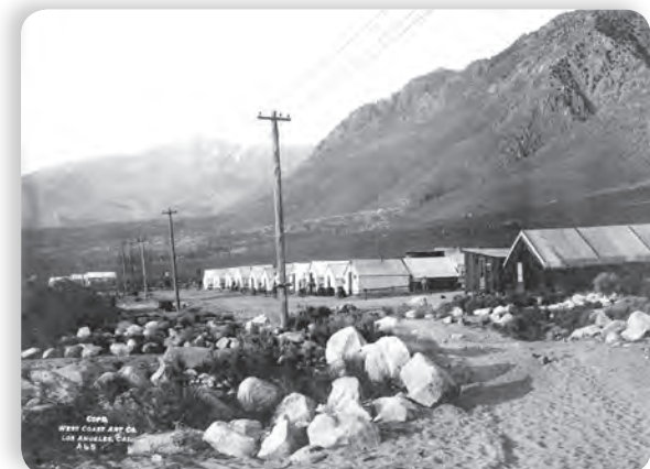
Construction Camp in Olancho Division, near Independence in the Owens Valley, 1911.
