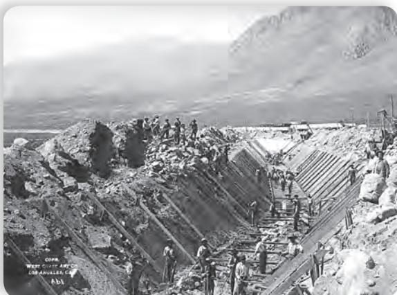
Lining the conduit with concrete in Olancho Division, near Independence in the Owens Valley, 1911.
