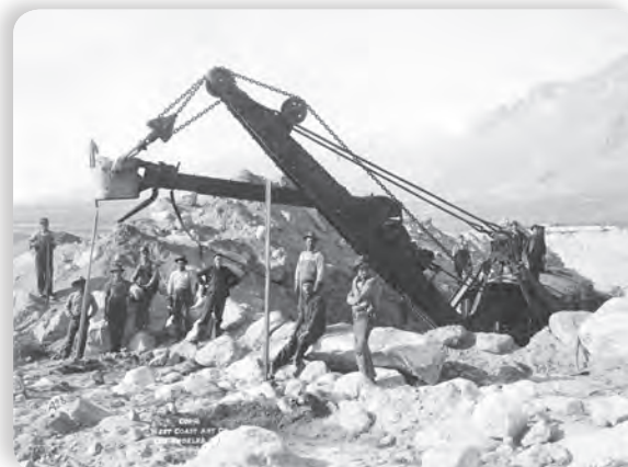
A steam shovel working in Boulders in Olancho Division, near Independence in the Owens Valley, 1911.
