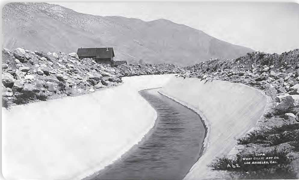
The finished aqueduct in Olancho Division, near Independence in the Owens Valley, 1911.
