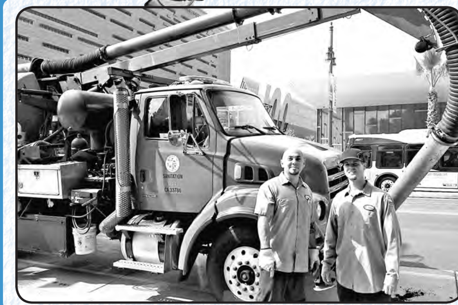
As discovered by Jackie Causillas, Club Counselor: Here are two workers from Public Works/Sanitation, hard at work on Main Street downtown. From left: Mike Bejarano , Wastewater Collection Worker II, 7 years of City service, and Robert Thuesen , Wastewater Collection Worker II, 5 years.
