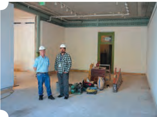
The inside of the Sepulveda Building during construction, June 2012. Pictured are (from left) Eric Hess, Sr. Construction Inspector, Public Works/Contract Administration, and Javier Gonzalez, Construction Manager, Public Works/Engineering.
