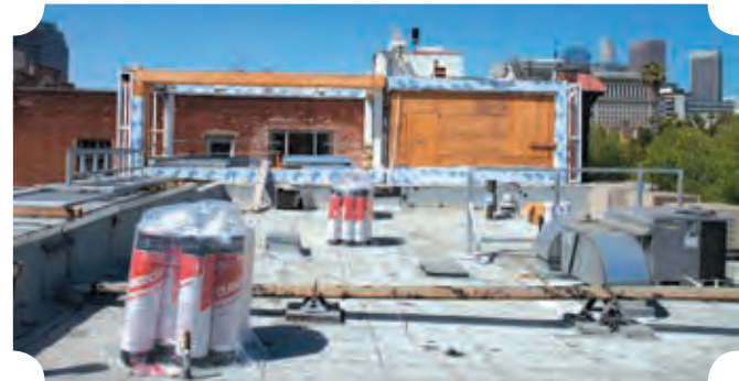
The viewing platform under construction.
