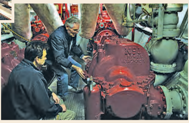
LEFT: Club CEO John Hawkins (left) and Fire Boat Pilot Bill Dahlquist, Retired, overlook a water cannon pump in the ship's engine room below the deck.
