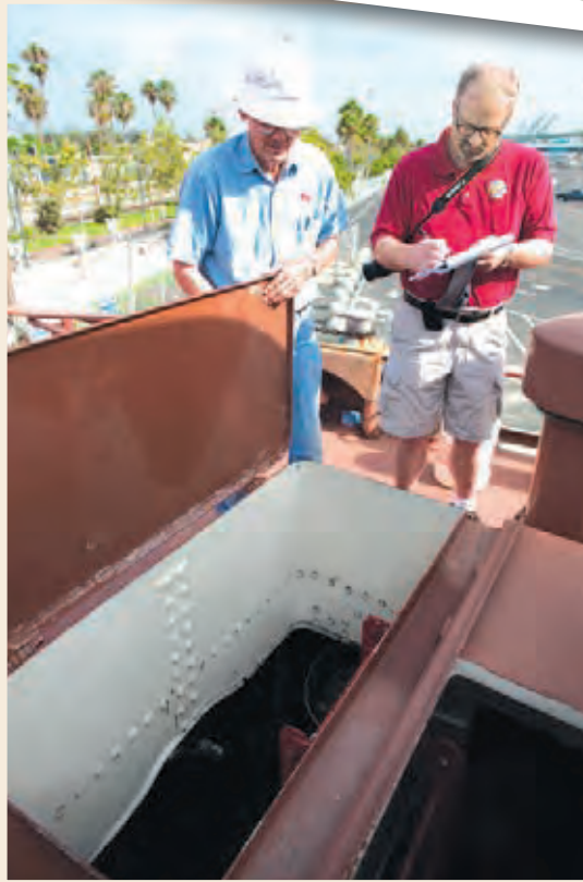
Bill Dahlquist at the escape hatch for the engine room and forward hold. "We're getting rid of the rainwater down there," he says.
