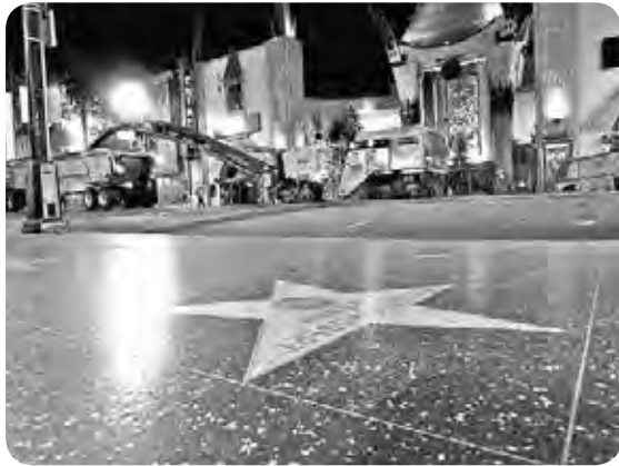
Street Services crews repave Hollywood Boulevard.
