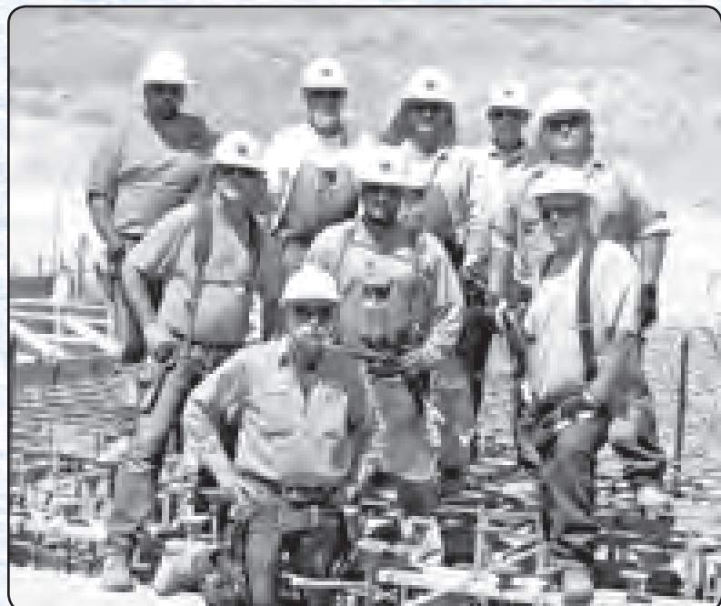
In the Owens Valley: Here's a DWP team building an irrigation distribution turnout station for water operations on Owens Lake. The team pictured is comprised of the concrete crews from Owens Lake Construction and the Mojave Construction Yards. They are, front row: Norm Harris, Building Repairer . Middle, from left: Jake Emory, Building Repairer ; Marin Parra, Reinforcing Steel Worker ; and Dave Borchert, Building Repairer . Back: James McMurry, Maintenance and Construction Helper ; Todd Emory, Building Repairer ; Ian Greer, Maintenance and Construction Helper ; Robert Turner, Construction and Maintenance Supervisor ; and Jerry Ross, Maintenance and Construction Helper . Special thanks to Larry Patrich, Construction and Maintenance Supervisor, DWP, Club Member, for sending us the photo.
