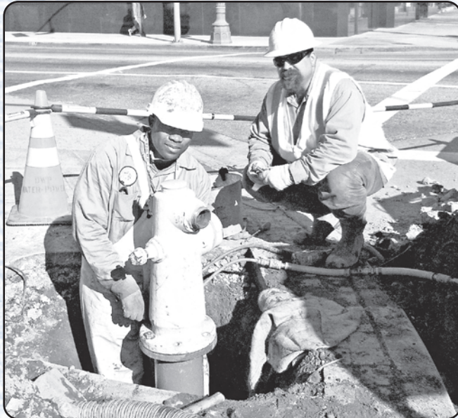
Repairing a fire hydrant at Second and Spring Street downtown are, from left: Tommy Gibbs , Water Utility Worker, 14 years of City service; and Vernon Chesterton, Sr. , Water Utility Worker, 8 years.
