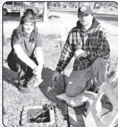
Here's a photo of Rec and Parks employees working on an irrigation system near the Cabrillo Marine Aquarium in San Pedro. From left: Traci Rubner, Sr. Gardner, 9 years of City service; and Frank Holmes , Irrigation Specialist, 1 year.
