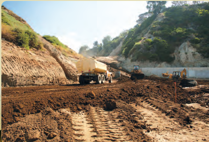
ABOVE: Many hundreds of thousands of cubic yards of dirt will need to be moved on the Potrero Canyon Project.
