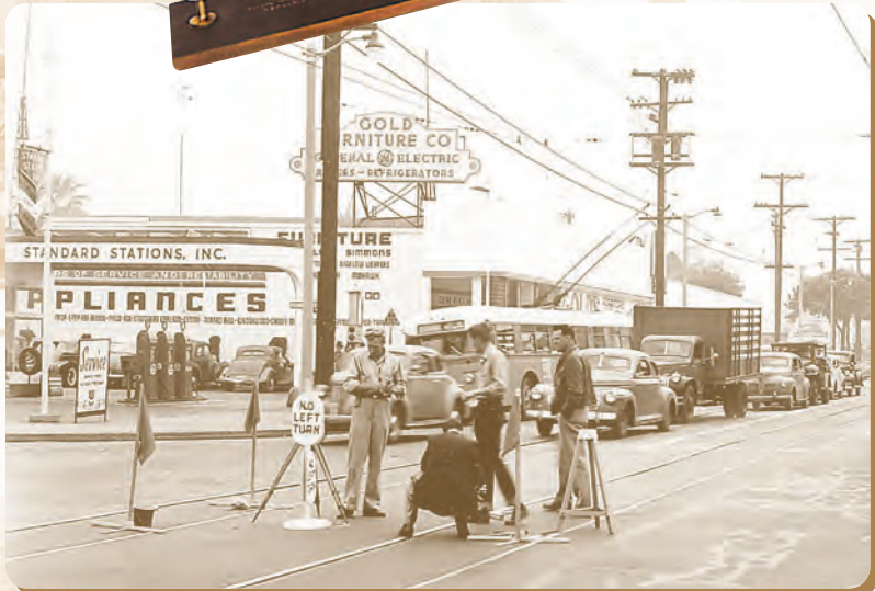
City survey crew establishing the center line intersection of the streets. A cast iron monument cap, still in use today, is seen at the left and is anchoring the "homemade" traffic safety flag.
