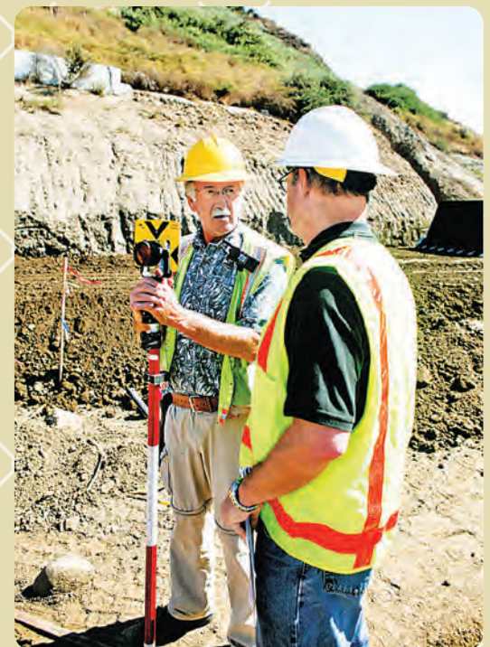
ABOVE: Rick Allen, Field Engineering Aide, 25 years of City service, explains the surveying portion of the Potrero Canyon Slope Stabilization Project to Alive! editor John Burnes.
