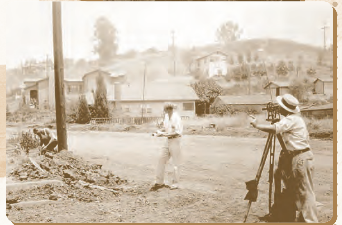
City survey crew providing staking for new curbs.
