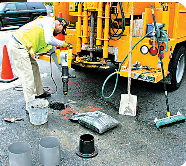
ABOVE: A Survey Division drill rig crew installs a monument into a City street.
