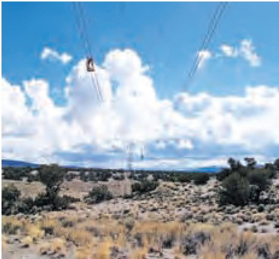
"This picture was taken above Benton during our October SIR (outage) of the Sylmar-Cililo DC line. It is Ben Rodriguez (Club Member) spacing from a cart."
