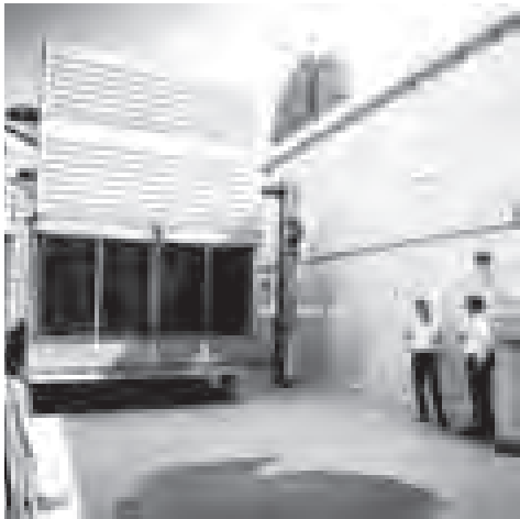
Rey Castro (right) displays the Convention Center's efficient chillers to Club CEO John Hawkins.
