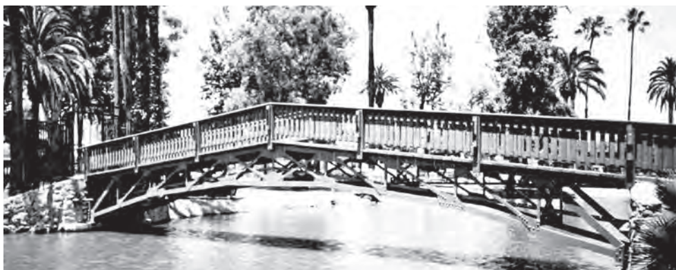
The Echo Park Bridge, restored to its original glory.
