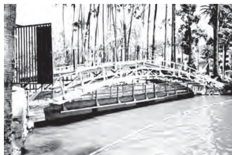
Scaffolding is up on both sides of the bridge, which is ready for rebuilding.
