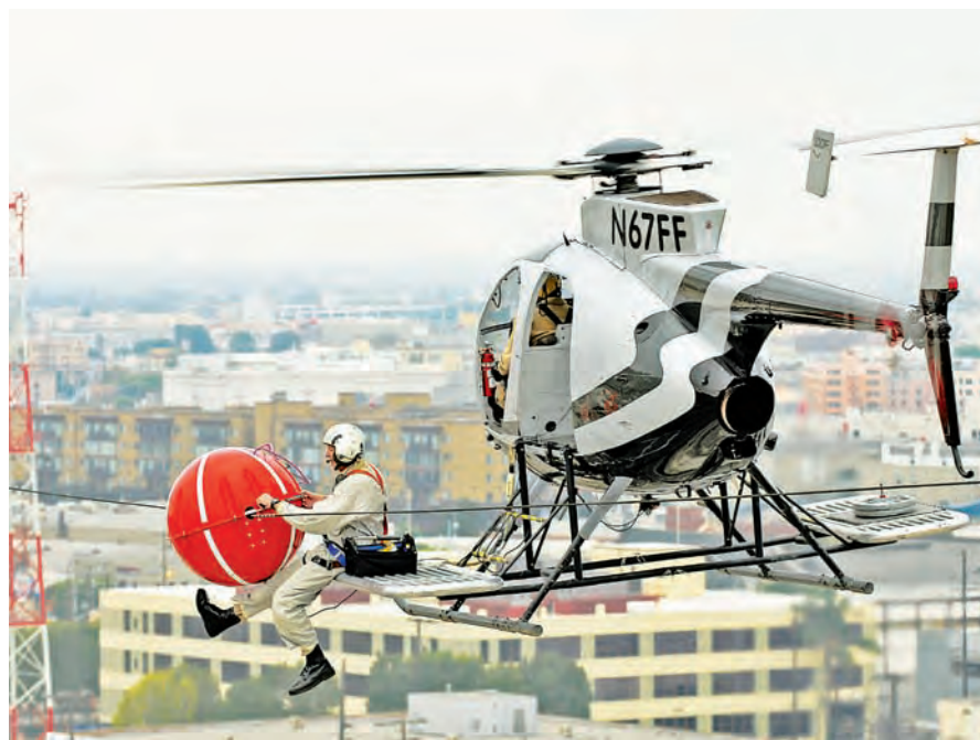
"This photo is of a lineman installing aircraft marker balls on the DWP's transmission static lines above an energized 230kv circuit that runs along the L.A. River across from Piper Tech. I was on the tower about 100 feet north of them. Taken on Oct. 11."
