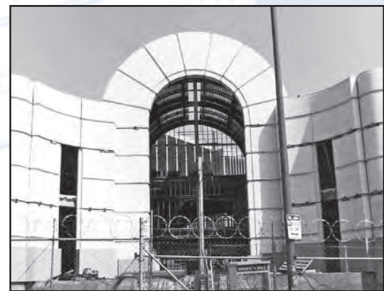
The L.A. Chamber of Commerce building at 350 S. Bixel St., under construction in April 1994.
