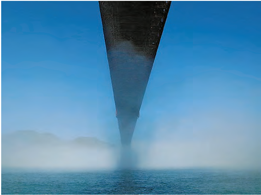
"Through the fog, at the Golden Gate Bridge." - Mike Aubin, Airports
