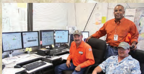
From left: Gary Reiser, Aqueduct and Reservoir Keeper; David Neal, Operations Manager; and Larry Benbrook, Aqueduct and Reservoir Supervisor, in the current SCADA (Supervisory Control And Data Acquisition) room.
