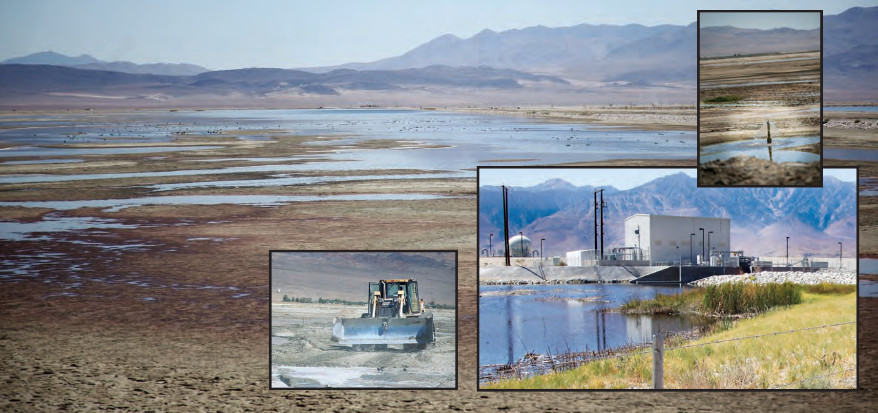
A dozer clears a flood channel (left), the pumping station at the end of the Lower Owens River (middle); a bubbler is used to distribute the water (right).
