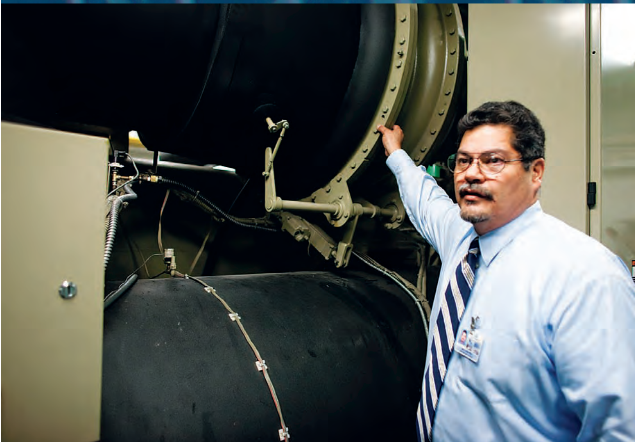
Rey Castro explains a point about the Convention Center's water chiller system.
