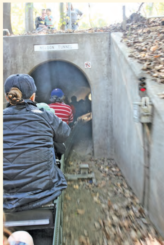
The Nelson Tunnel.
