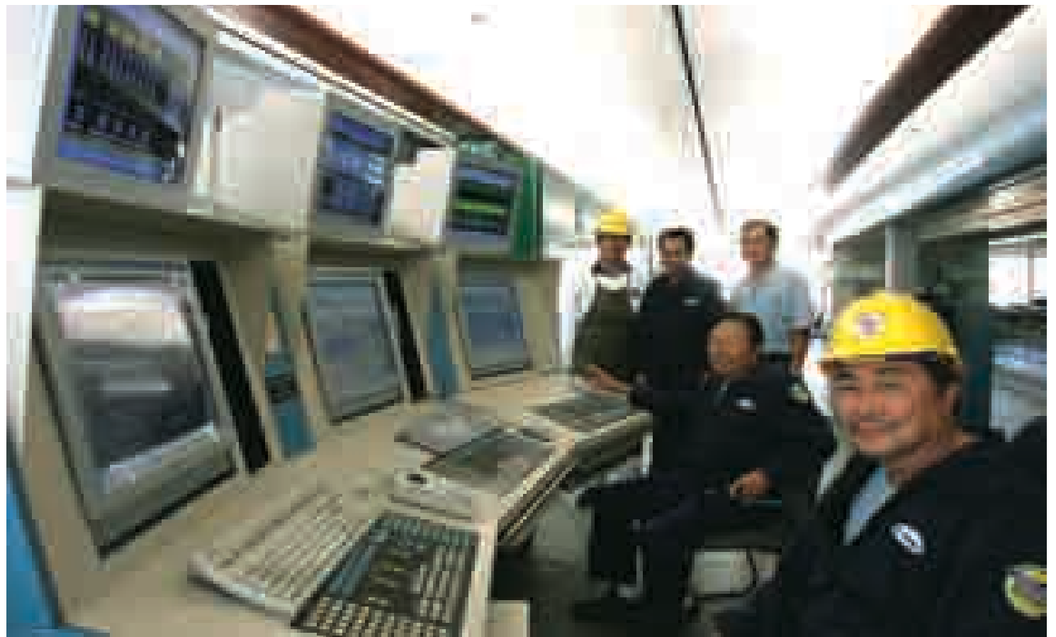
At the Secondary Treatment Operations Center Control Room are, back row, from left: Chang Huang, Instrument Mechanic, 18 years; Rudy Lingat, Waste Water Treatment Operator I, 20 years; and Allan Huang, Waste Water Treatment Operator II, 23 years. Seated: Serafin Malabanan, 17 years, and Oscar Espineda, Waster Water Operator, 22 years.
