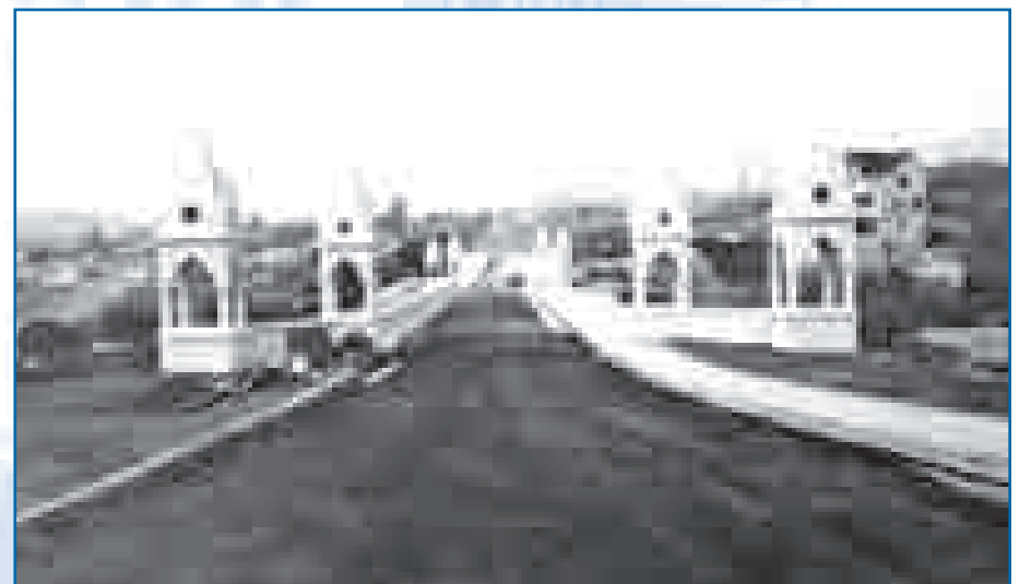
The Franklin Avenue Bridge.
