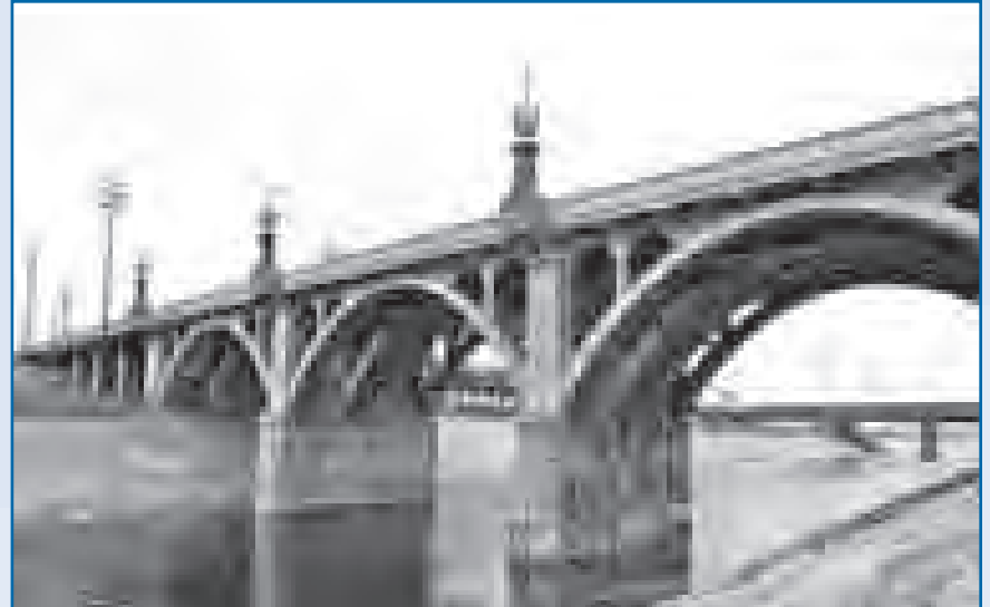
The Olympic Street (Ninth Street) Bridge.
