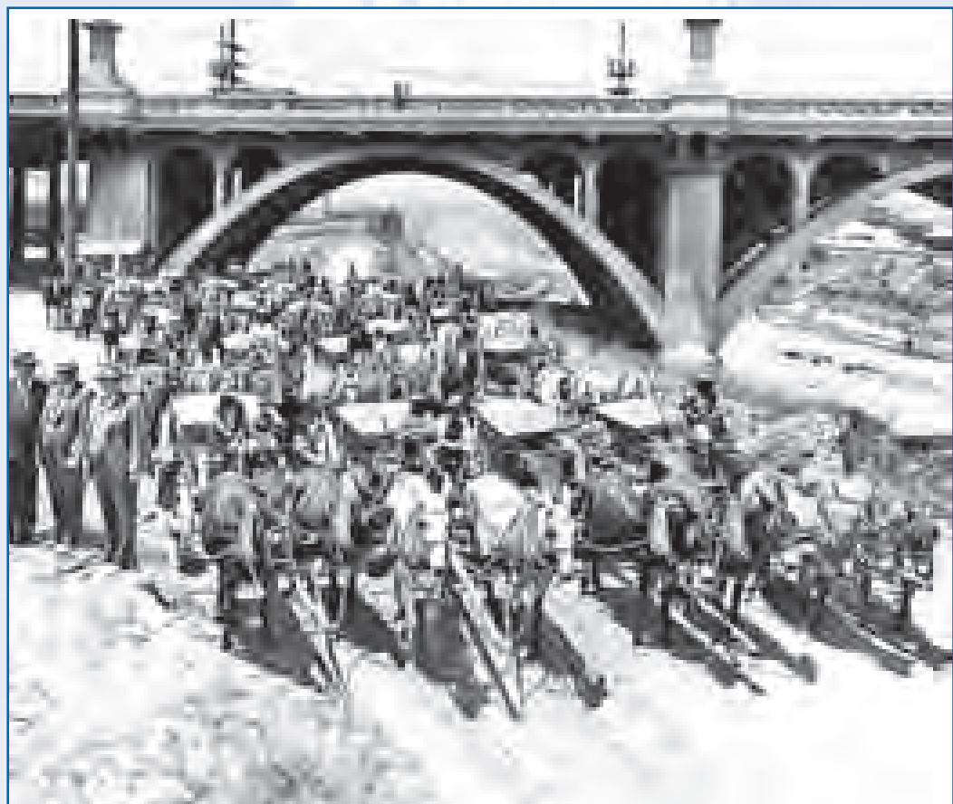
The (then) Ninth Street Viaduct under construction circa 1925. Work was being done by the North Pacific Construction Co.
