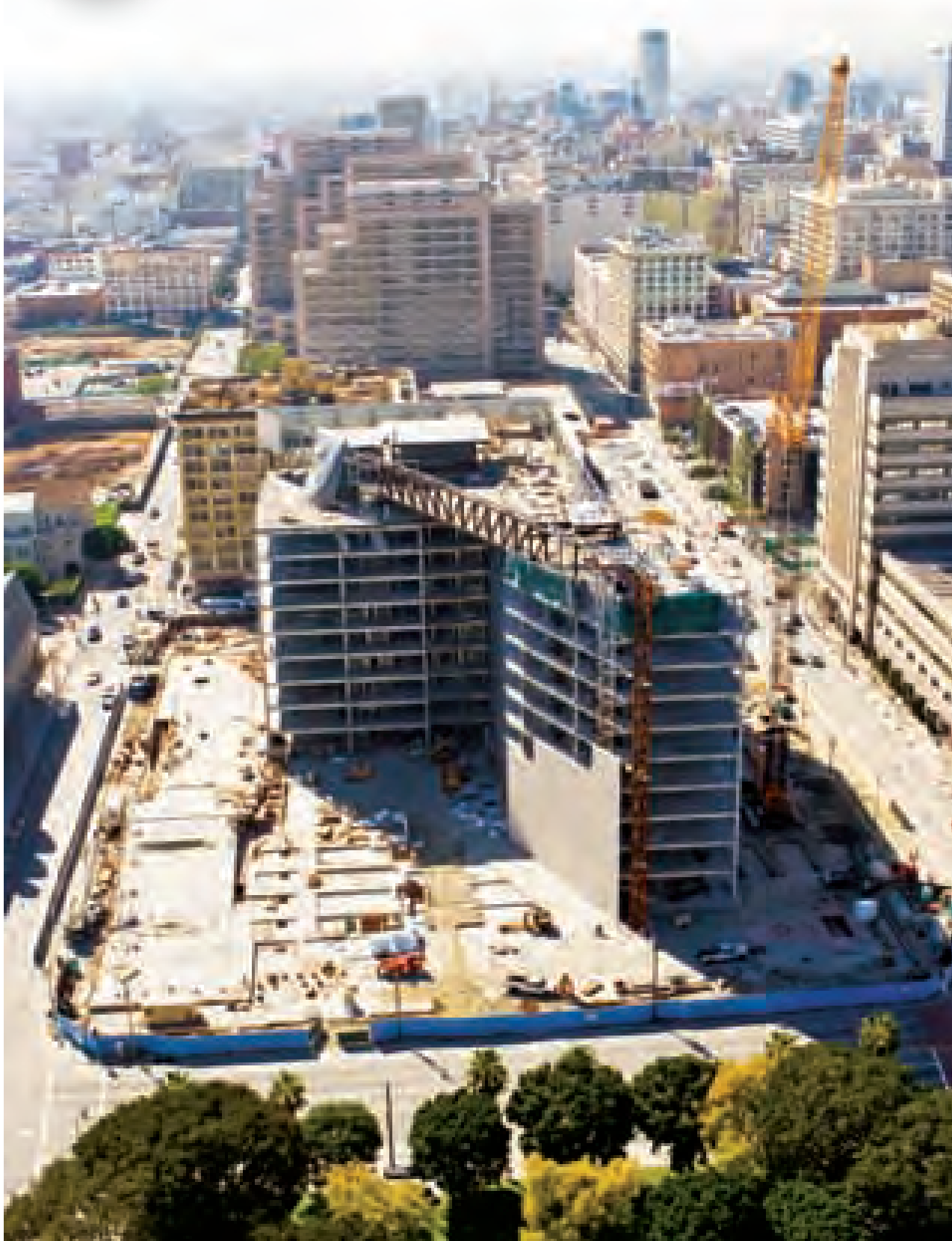
This photo by Club Tech Guru Summy Lam from the top of City Hall, shows the new Parker Center's construction progress.
