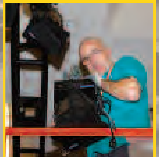
BELOW: Mark Skelly, Electrician.
