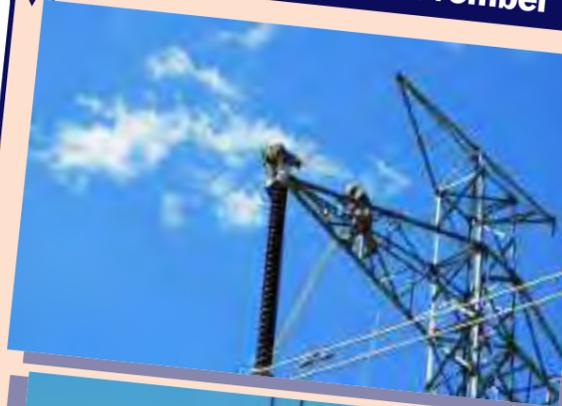
"Cooning the bells -- This tower is 135 feet tall. Cooning the bells means climbing down the insulators to the wire, then you put a spacing cart on. The spans are a quarter-mile long."
