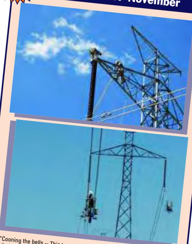
"Cooning the bells -- This tower is 135 feet tall. Cooning the bells means climbing down the insulators to the wire, then you put a spacing cart on. The spans are a quarter-mile long."
