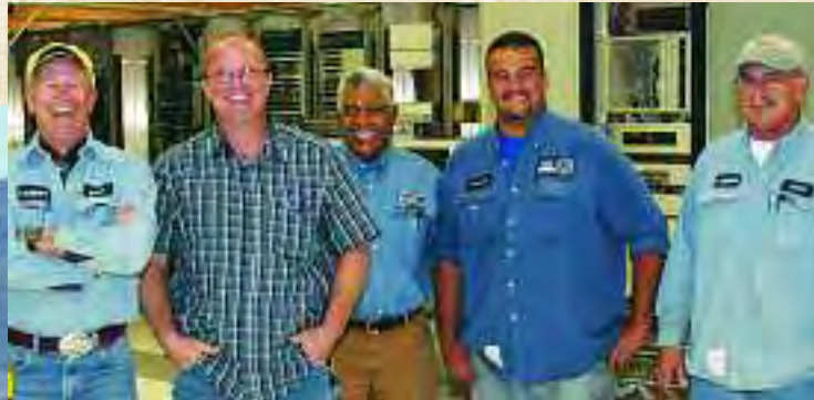
Performing a remote terminal upgrade at Marketplace are, from left: Mike Able, Electrical Mechanic; Al Derlighter, Electrical Mechanic Supervisor; Walter Johnson, Electrical Mechanic, Alfredo Cardenas, Electrical Craft Helper; and Vic Aceves, Electrical Mechanic.
