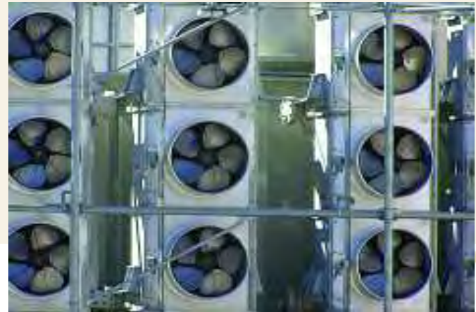
State of the art equipment converts DC to AC current and vice-a-versa.
