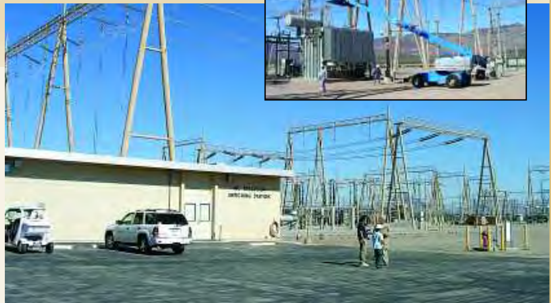
The McCullough Switching Station, south of Boulder City, gathers power from a number of sources and sends it where it's needed. Inset: Larry Jurn, Electrical Mechanic, is in the "bucket," installing a new transformer.
