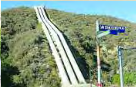
View of waterline.
