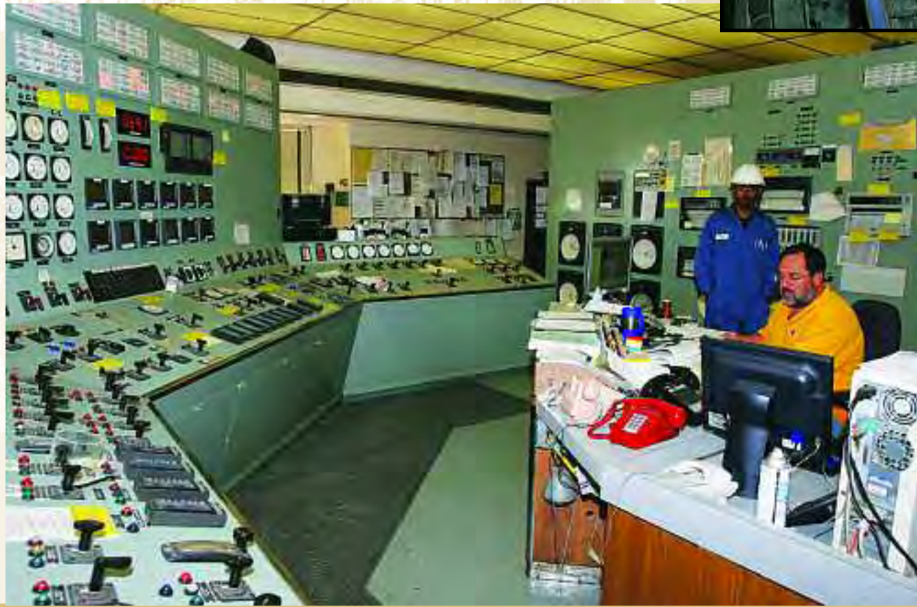
The Operator Control Room.
