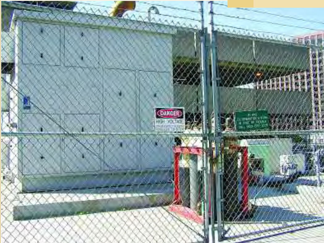
The fuel cell at the John Ferraro Office Building.
