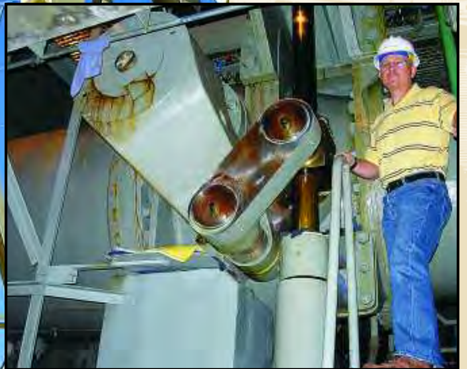
Water from the Los Angeles Aqueduct enters the Control Gorge Station via this penstock and valve. Standing next to it is Jeff Husted, Chief Electric Plant Operator.
