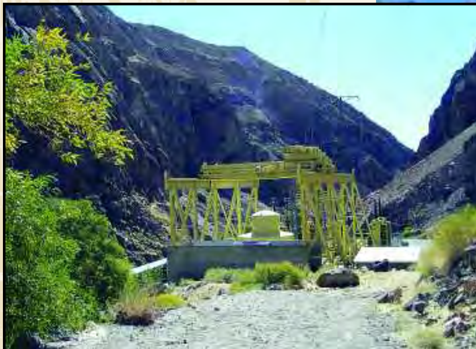
Middle Gorge Generating Station is not staffed.
