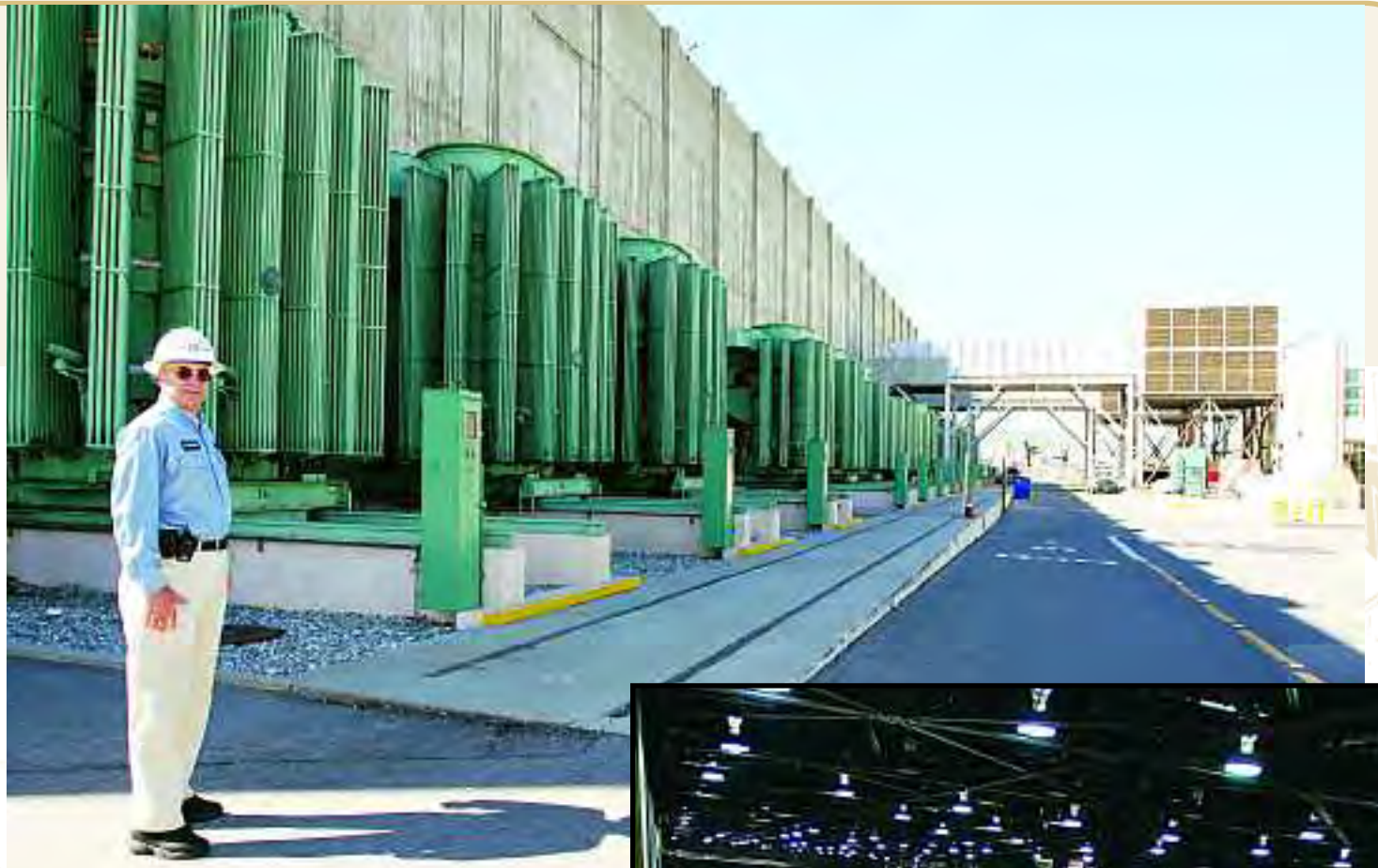
Mostafa Haji, Plant Engineer, 18 years of service, at the Harbor Generating Station.
