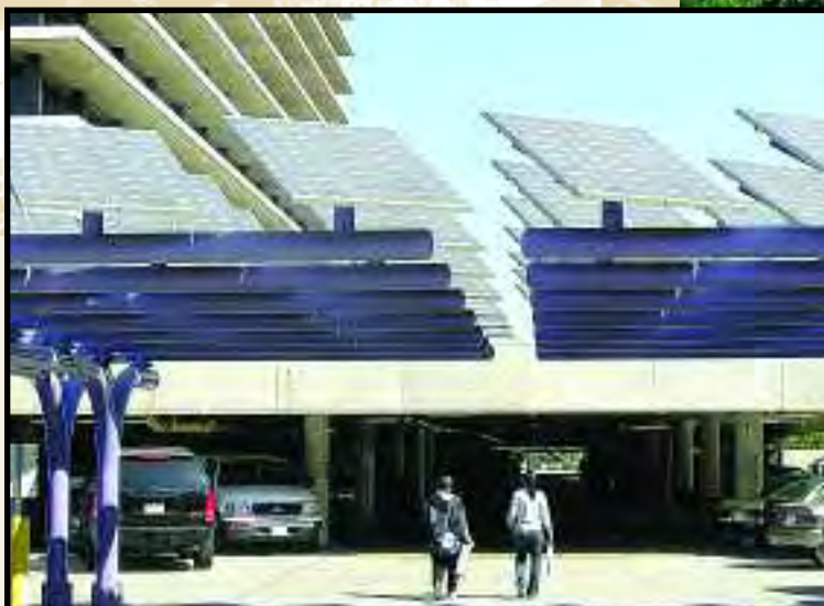
Solar arrays at the John Ferraro Office Building.
