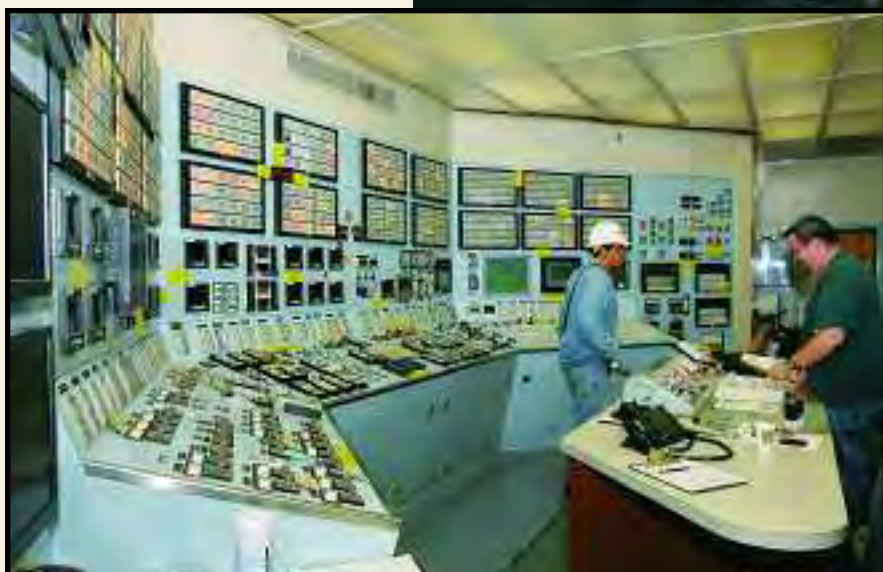
Control room for the generating station.
