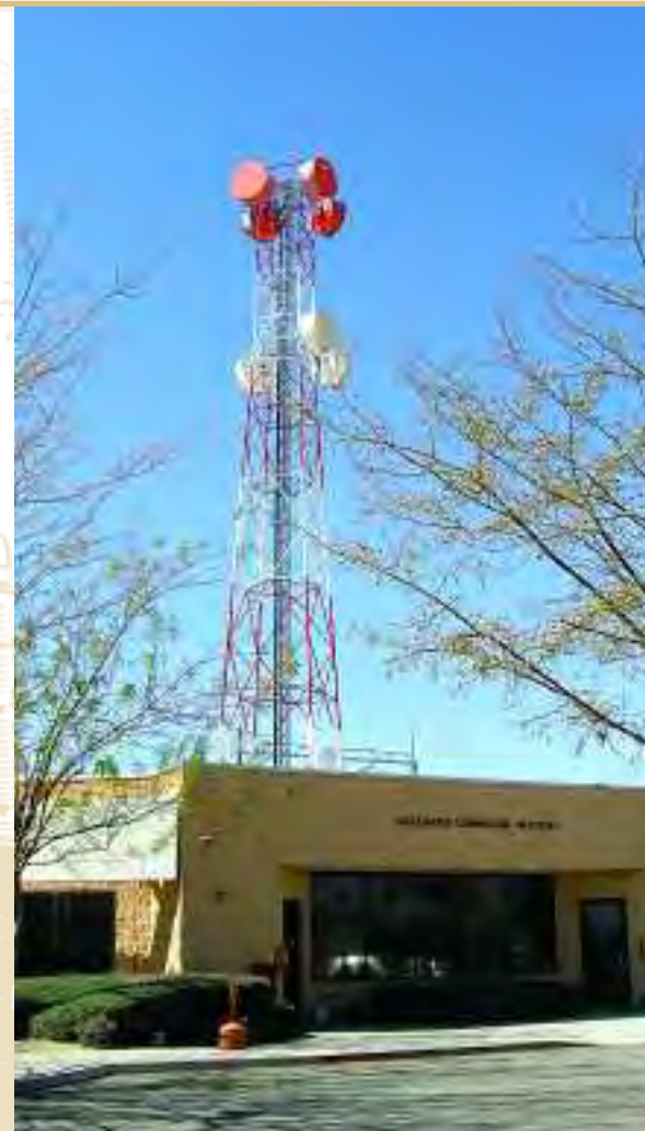
The Adelanto Converter Station in Adelanto, near Victorville. A microwave tower soars above it.
