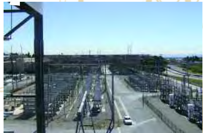
The Sylmar converter station has stood the test of earthquakes over the decades.
