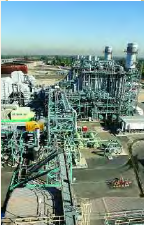
View from top of Haynes Generating Station.
