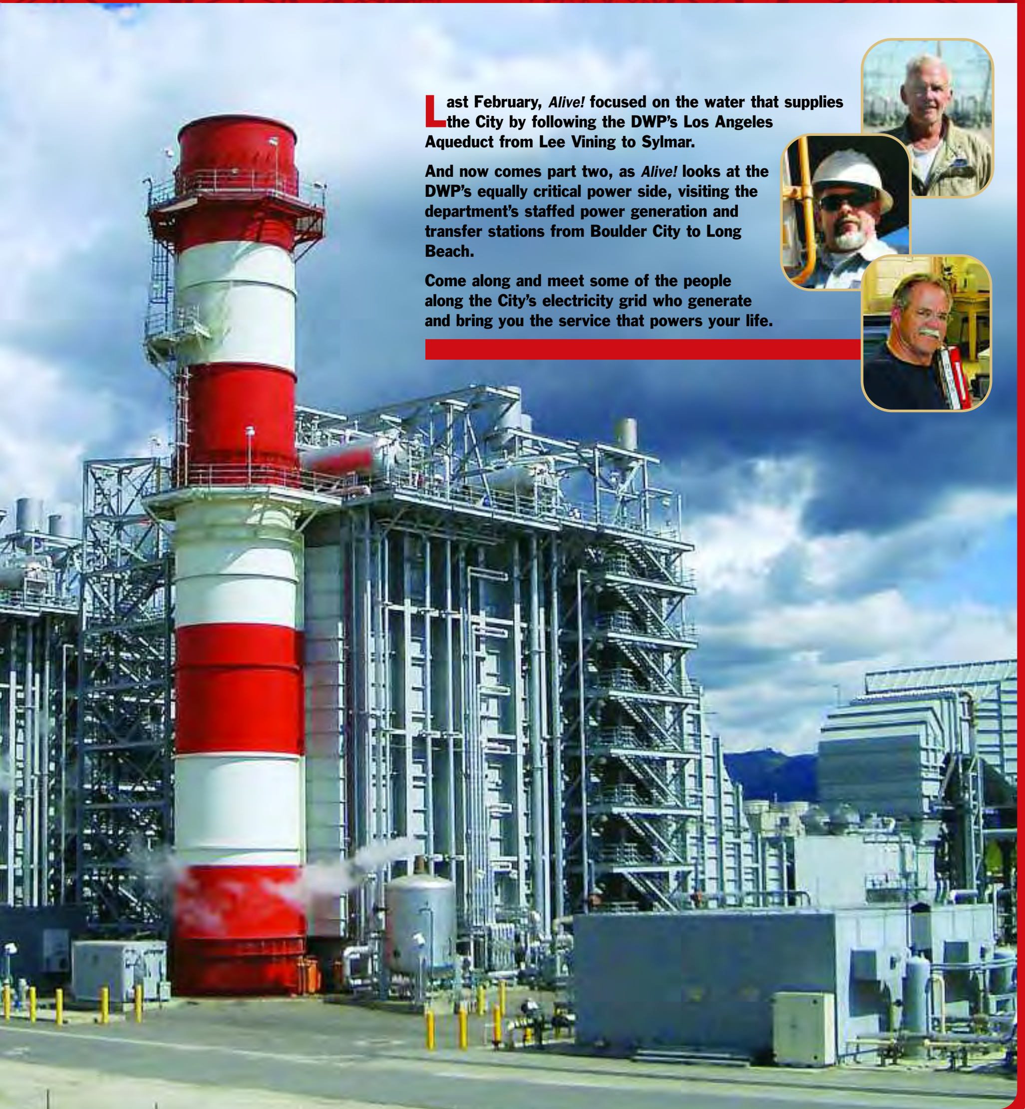
Valley Generating Station photo courtesy DWP
