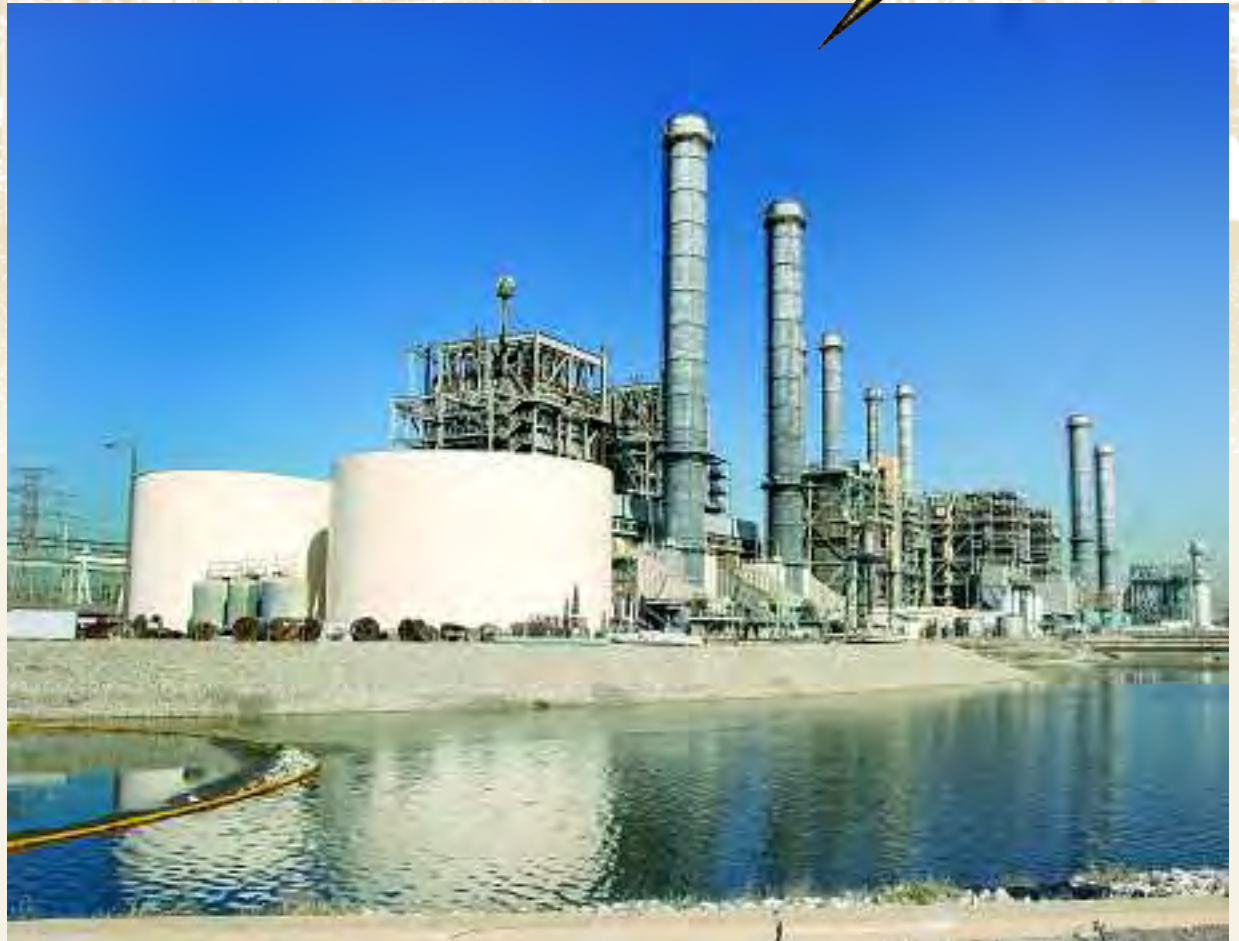
Generating Station landscape from the front of the plant.
