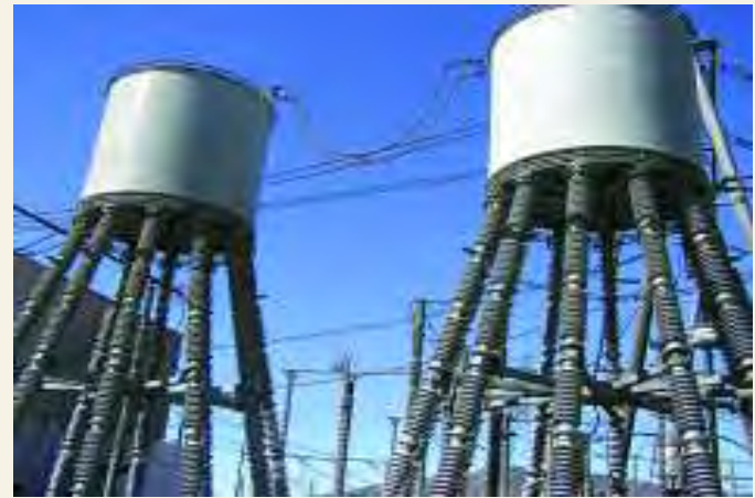
Smoothing reactors work like a resistor and limit current.
