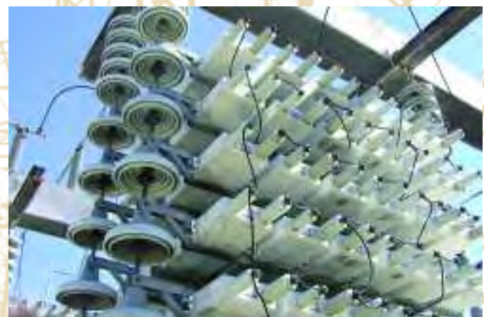
DC filters have to be cleaned every other year since the electricity collects dust onto the surface of equipment.
