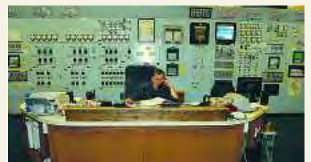
Another control room for the generating station.
