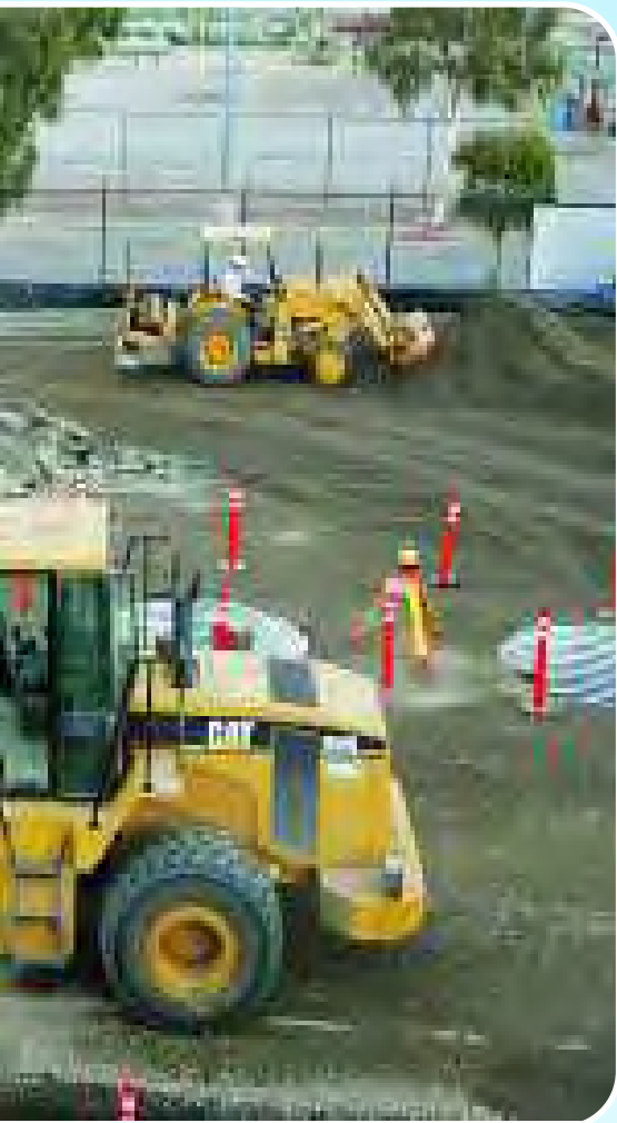
Workers have started digging the two mile-deep holes that are critical to the T.I.R.E. Project.
