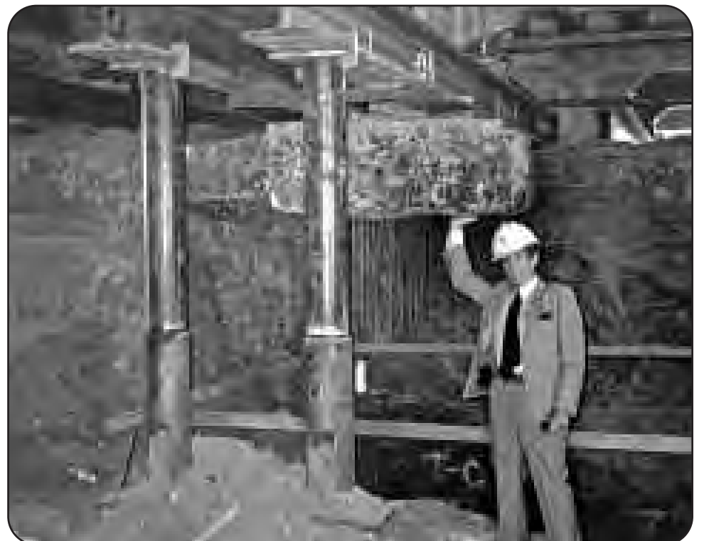
Dr. Ed Krupp pretends to be Atlas in "holding up" the old support beams during the excavation of the new Observatory space, under the building's front lawn. New support beams were put in to accommodate the expansion.
