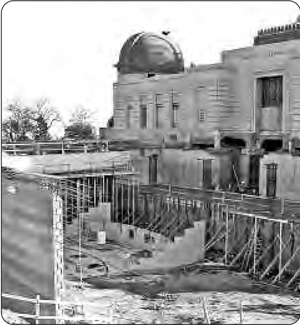
The front lawn of the Griffith Observatory was dug up temporarily to construct a major expansion underground. The lawn has since been restored. The beginning of the Leonard Nimoy Event Horizon Theater can be seen.
