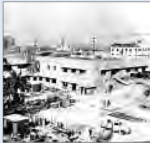
The current Central Receiving Hospital under construction in 1956. The hospital is scheduled to be razed.
