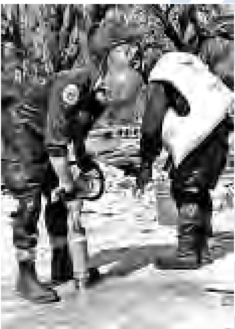
LAFD Tech Search Specialists and USAR Team Members Patrick Leising and Jerimia Spring at work in Mississippi. Patrick uses a Pomeroy to cut an access hole for the search cam. Jerimia uses a water pack to control the concrete dust.
