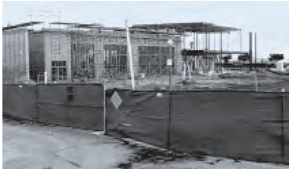
The new Fire Station 5 is under construction (above) in Westchester. The new station, one of 20 new LAFD stations, is scheduled to open in March 2006.
