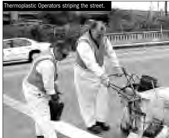
Thermoplastic Operators striping the street.
