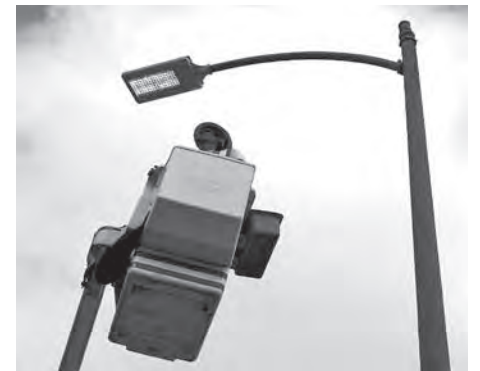
Public Works/Street Lighting's Tim Spradley inspects an LED light being tested.
